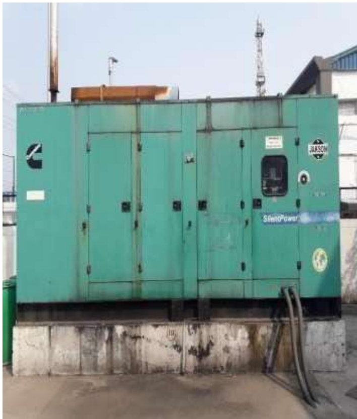
380-KVA CUMMINS GENERATOR
